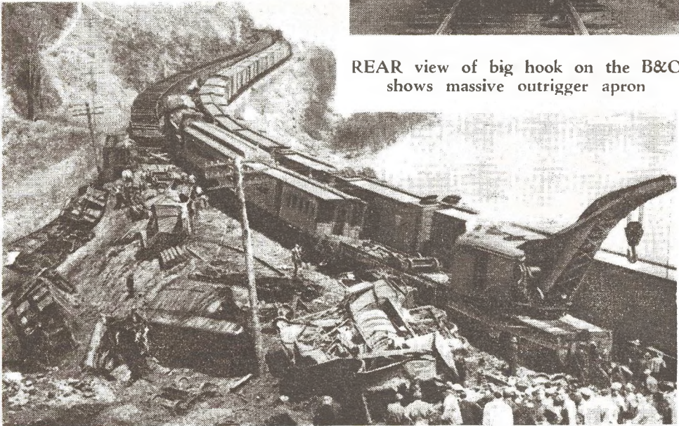
OPEN switch threw a Lehigh Valley coal train into a string of empties at Lehigh, Pa., in 1934. The wrecker eased into position on track the overturned freight should have taken
