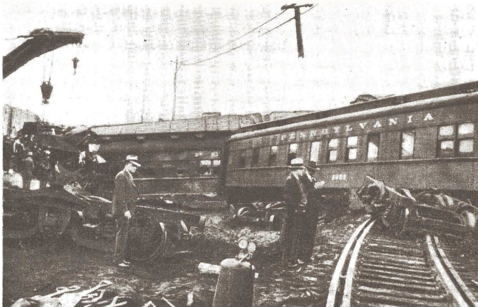
TELEGRAPH poles hung like kite frames from their wires when excessive speed on a sharp curve caused this wreck at Minson, N. J. (See Item 4)
