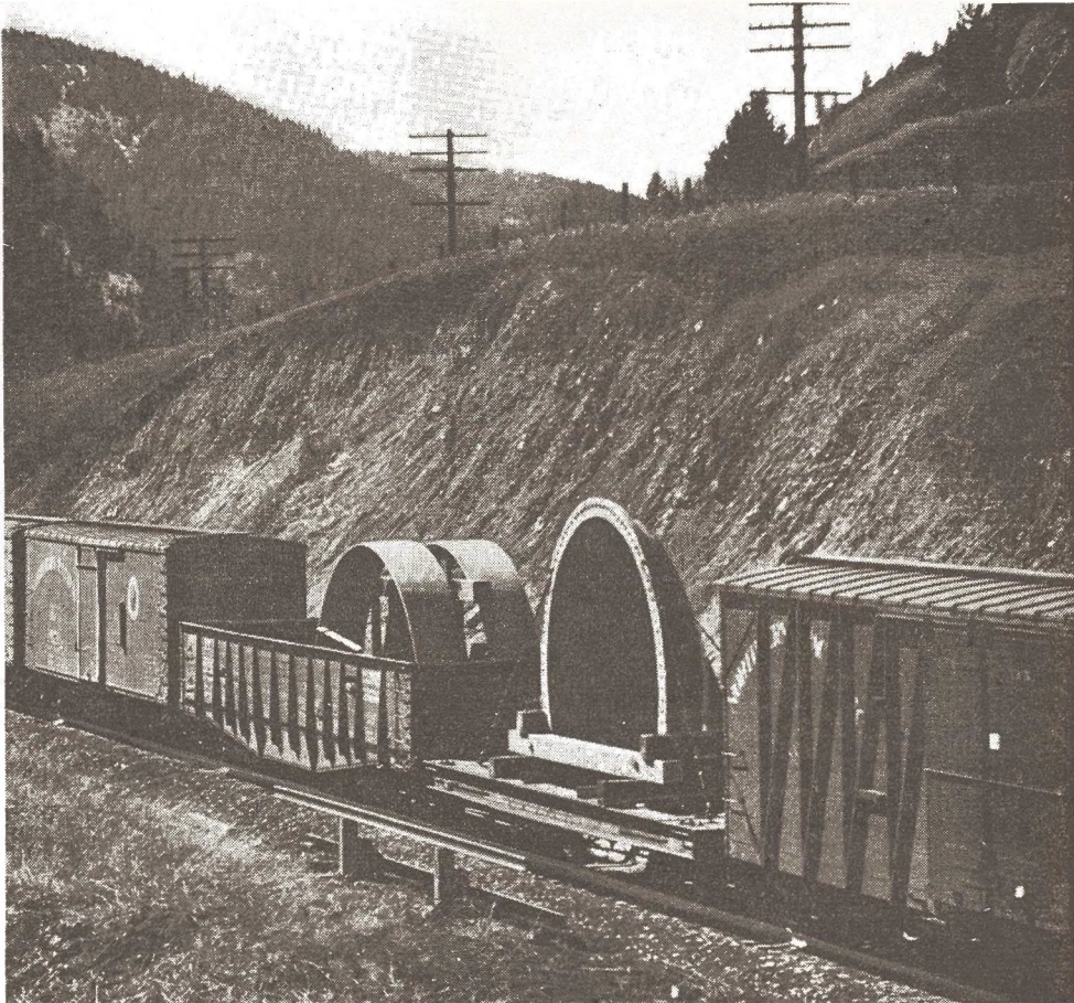
BOUND for a hydro-electric project, oversize shipments thread Rocky Canyon toward Northern Pacific's Bozeman Pass. As a rule such consignments are placed near the engine, where they are under constant surveyance
